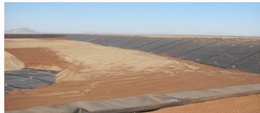
Tailing Impoundment Sand Liner – final step
