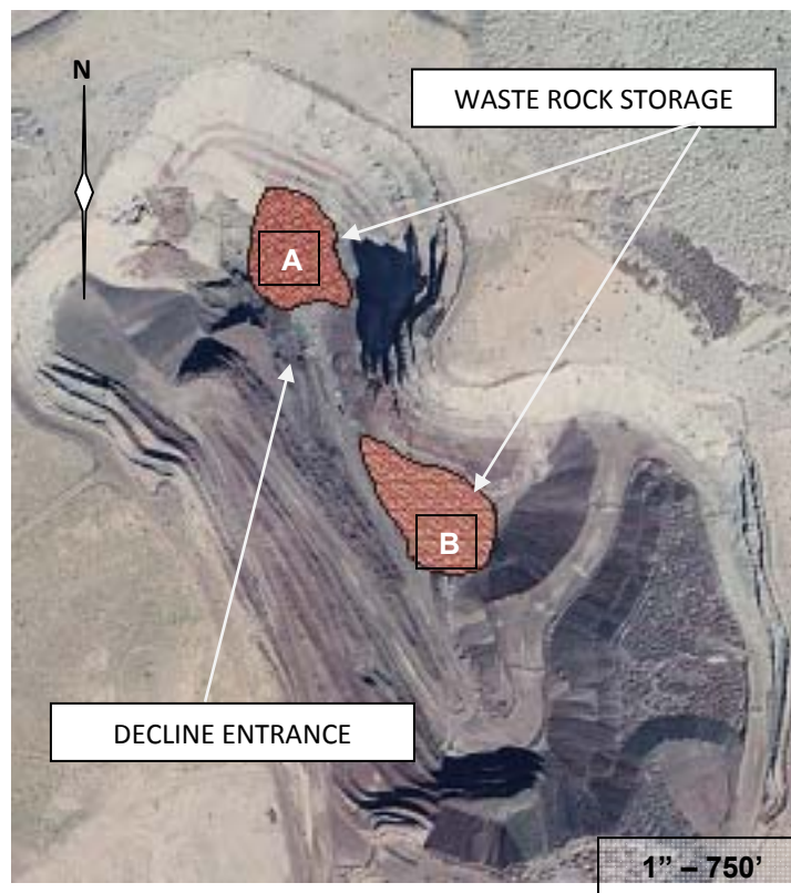
Figure 18-1: Waste Rock Storage Areas
