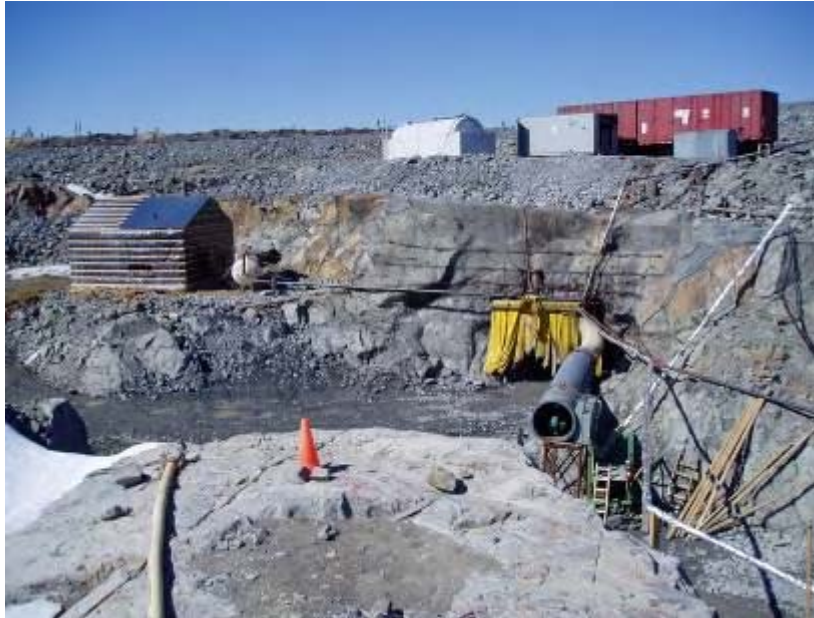
Figure 9 – Ramp portal in the north wall of the pit.
