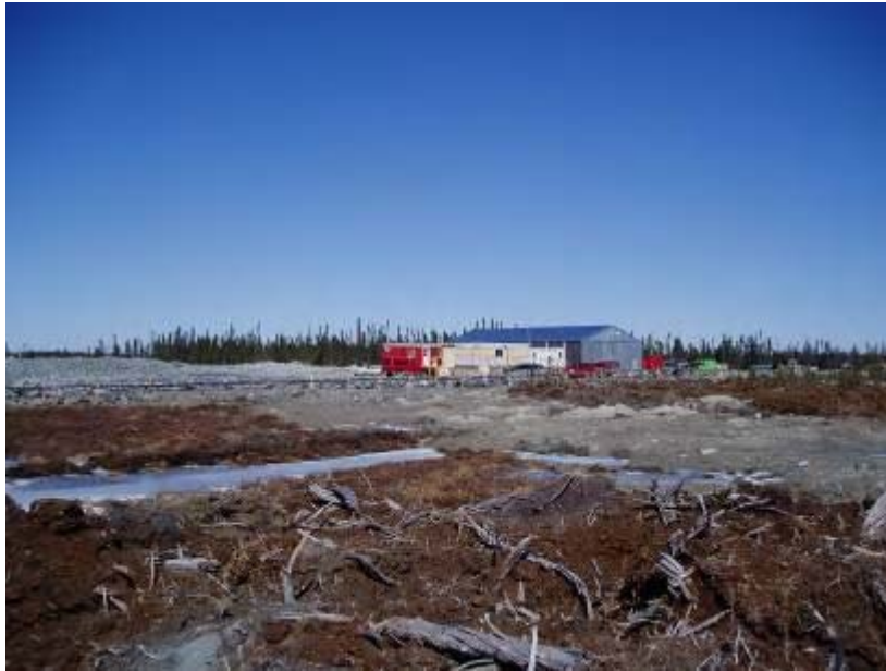
Figure 4 – Project facilities: technical office and garage in August 2004.
